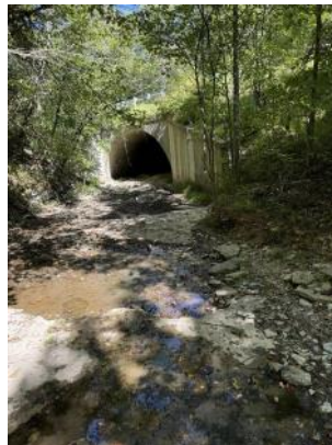
Tunnel under Highway 50 ride
